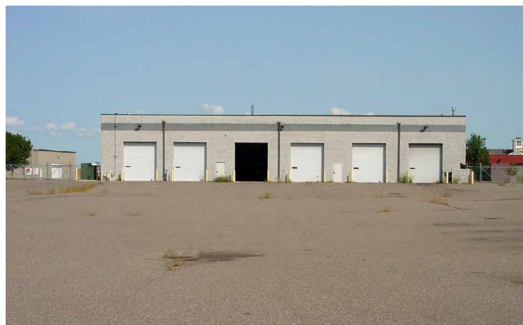
REAR OF MAIN BUILDING
